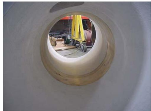
The same view after rehabilitation work is completed. Note the smooth unblemished wall surfaces, clear of scale, corrosion and defect along with clean throat region. The internal geometry has been precisely surveyed, recorded, and new flow calc provided.
